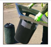
The Water Decontaminator Trash Capture series is a patented, environmental product that is placed under a catch basin grate to help remove trash, sediment, oil and contaminants from run off. Oil and contaminants are captured in a disposable cartridge. The absorber cartridge uses recycled waste products, essentially fighting pollution with pollution.
